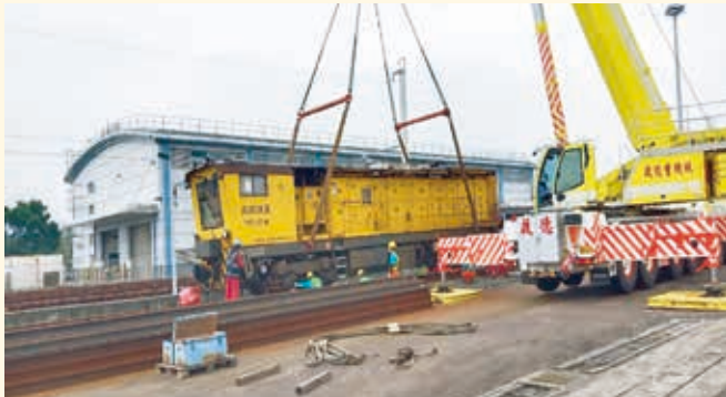
磨軌車吊掛作業 Rail grinding car hanging operation
