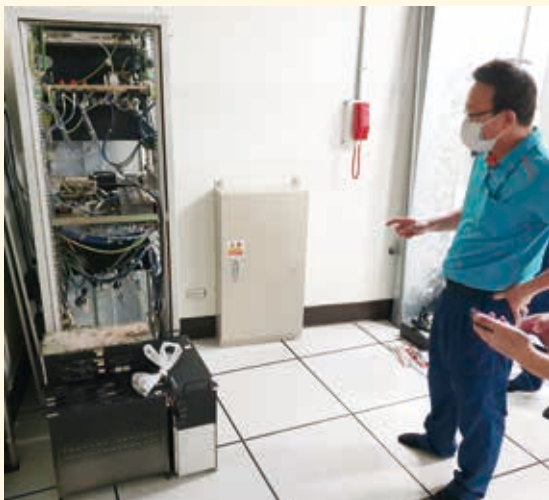
基地台拆移作業巡查 Base station demolition inspection
