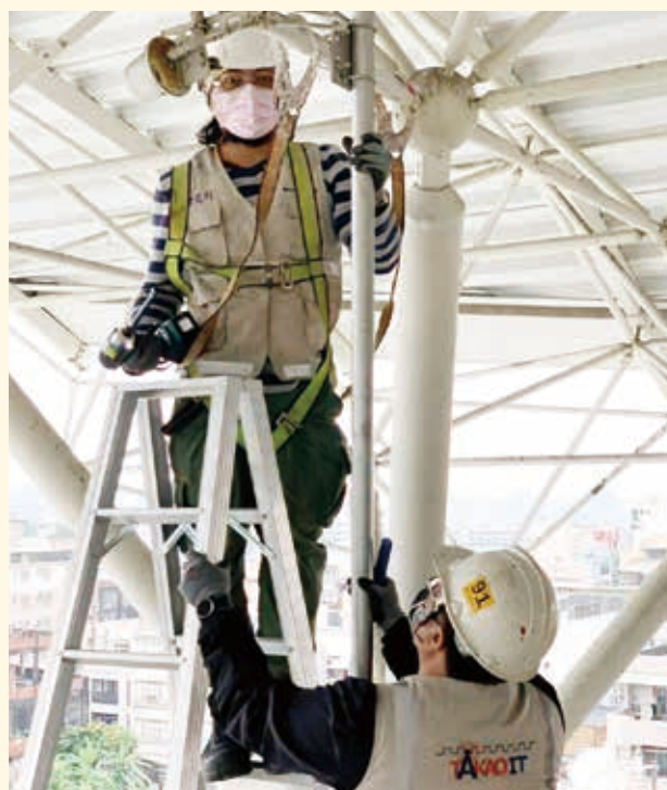
高架站天線移設 Elevated station antenna moving
