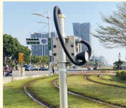
輕軌降噪系統現場安裝 Light Rail Transit Noise Reduction System On-site Installation
