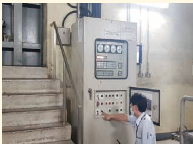
站務人員操作下放隧道防水隔艙閘門 Station staff operating the lower tunnel waterproof compartment gate
