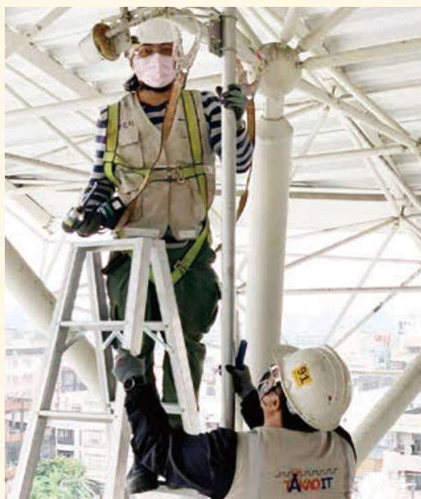
高架站天線移設 Elevated station antenna moving
